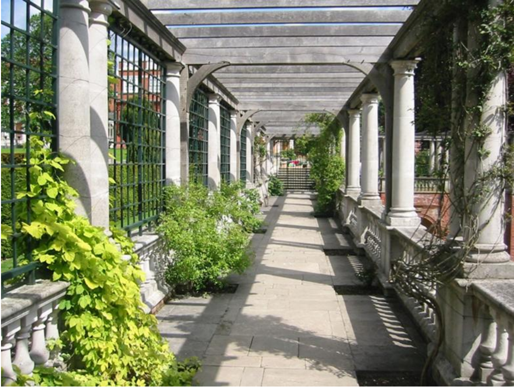
Section 1: showing upper level walkway with stone balusters and columns and planting beds which extend into the void between the paved surface and the structural slab.
