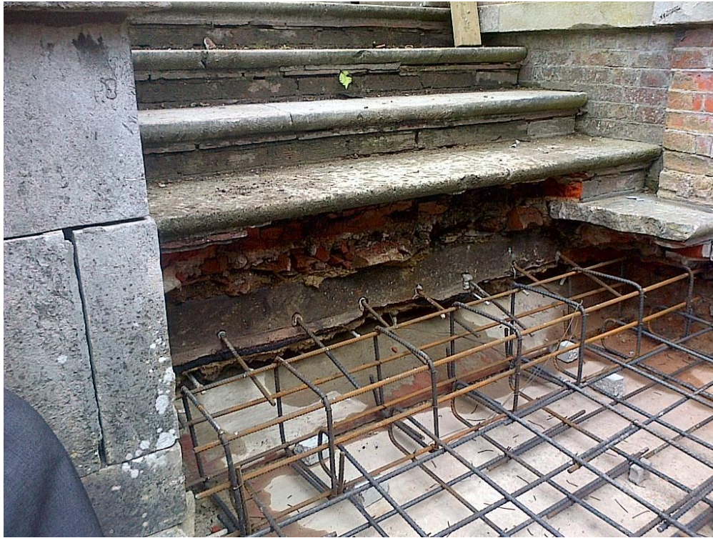
Section 2: repairs to Belvedere stair platform undertaken in 2014.
