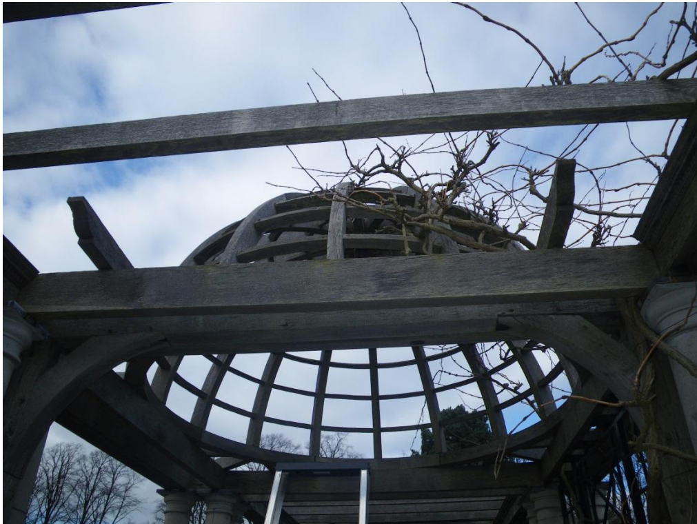
Section 1: dome shaped timber superstructure
