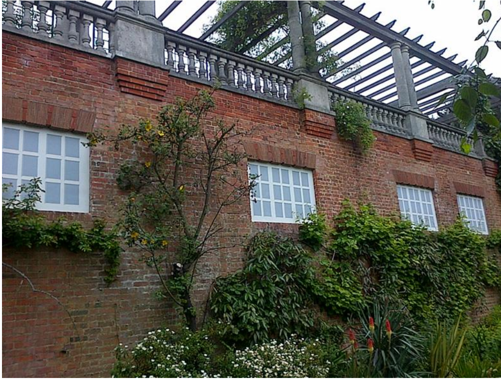
Section 2: The false windows after renovation in 2013.
