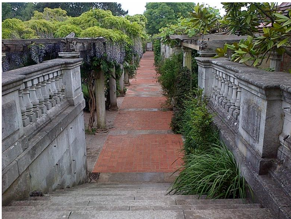
Section 2: general view showing renewed brick pavements.
