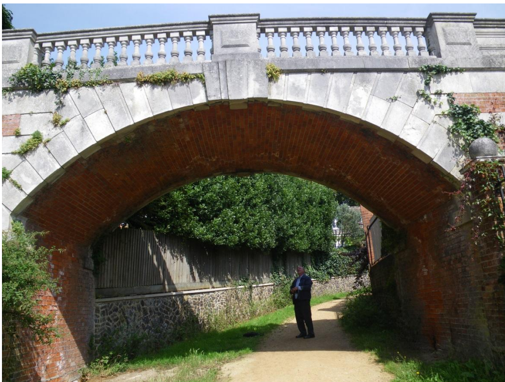
Section 2: The Bridge
